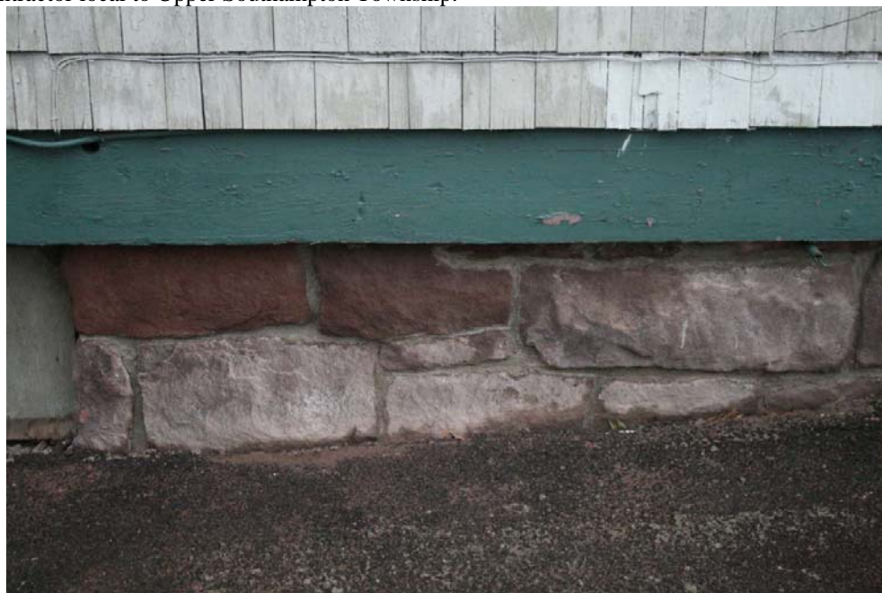
Restored building foundation, fall 2012
